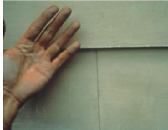
**FIGURE 6. Formation of fine powder on the surface of the paint film during weathering, can cause color fading. Although some degree of chalking is a normal, desirable way for a paint film to wear, excessive film erosion can result in heavy chalking.**
