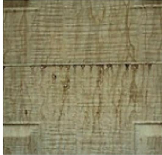
**FIGURE 7. Concentration of water-soluble ingredients on water-based paint, creating a blotchy, sometimes glossy appearance, often with a tan or brownish cast. More likely with tinted paints than with white or factory-colored paints.**
