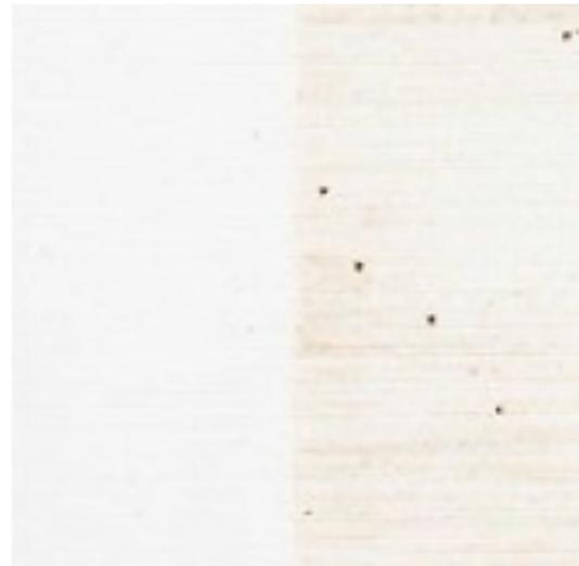
**FIGURE 14.** Brownish or tan discoloration on the paint surface due to migration of tannins from the substrate through the paint film. Typically occurs on 'staining timbers,' such as redwood, cedar and mahogany, or over painted knots in certain other timber species.
