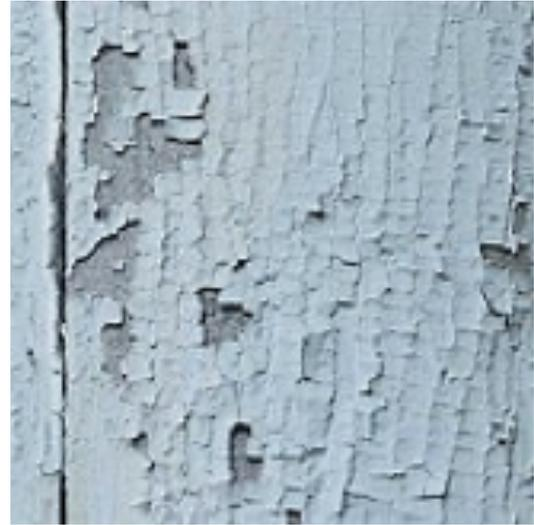
**FIGURE 3. Early on, the problem appears as hairline cracks; later, flaking of paint chips occurs. The splitting of a dry paint film through at least one coat leads to complete paint failure.**
